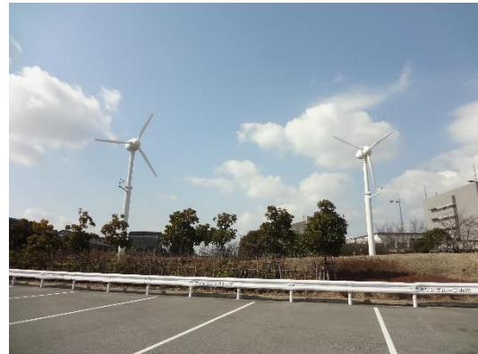
Wind power generation
