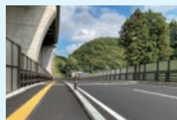
Railings to Block Discarded Objects
