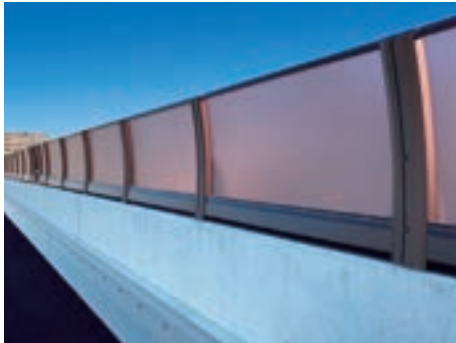
Railings to Block Discarded Objects
