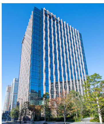
Sumitomo Fudosan Osaki Twin Bldg. East, Exterior
