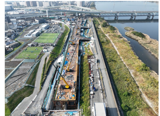
CM associated with embankment integrated road construction
